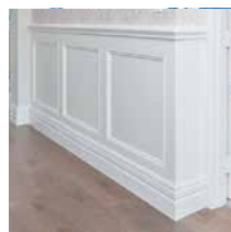
Skirting boards and primed wall panelling
