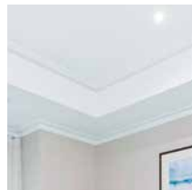
Feature ceiling recess to theatre
