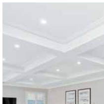
Feature ceiling recess to living area
