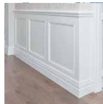
Skirting boards and primed wall panelling
