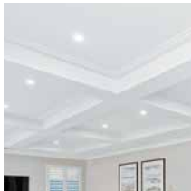
Feature ceiling recess to living area
